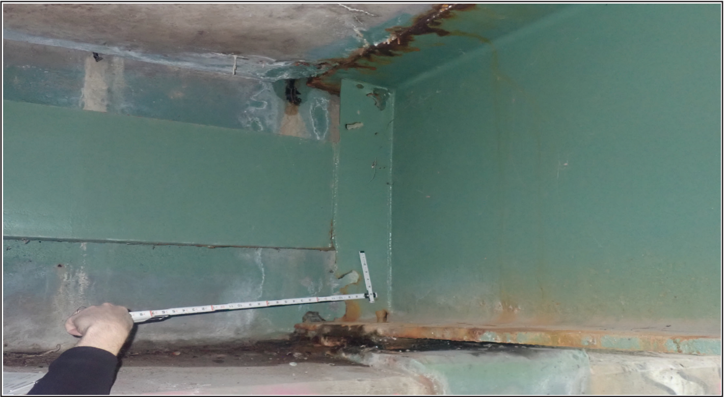
15 GIRDER 1 EXISTING PERFORATIONS IN STIFFNER OVER WEST BEARING
